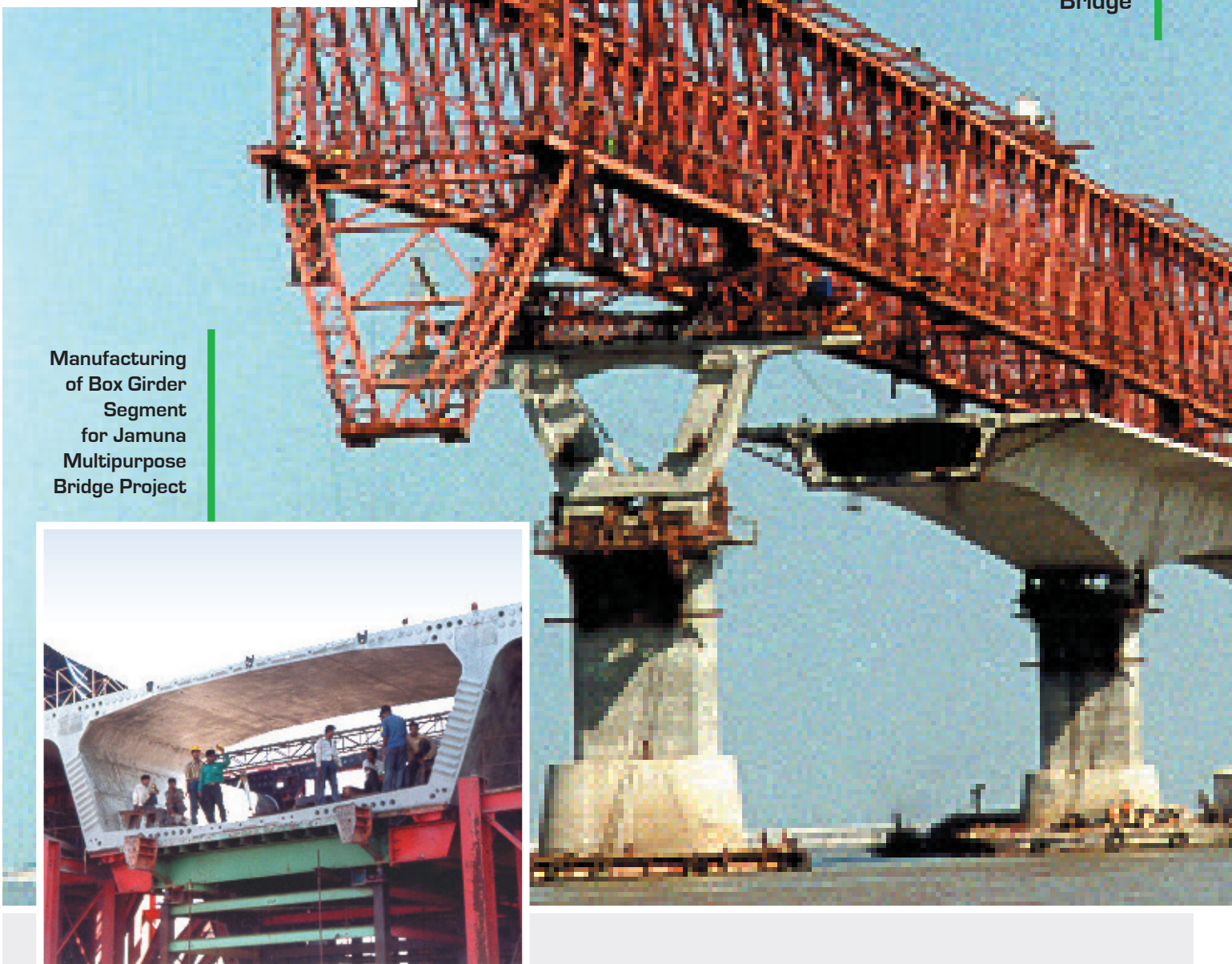
Installation of Box Girder Segment in Jamuna Multipurpose Bridge
