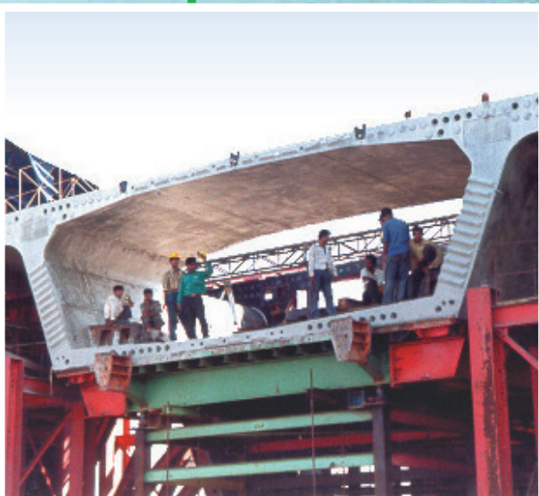
Manufacturing of Box Girder Segment for Jamuna Multipurpose Bridge Project
