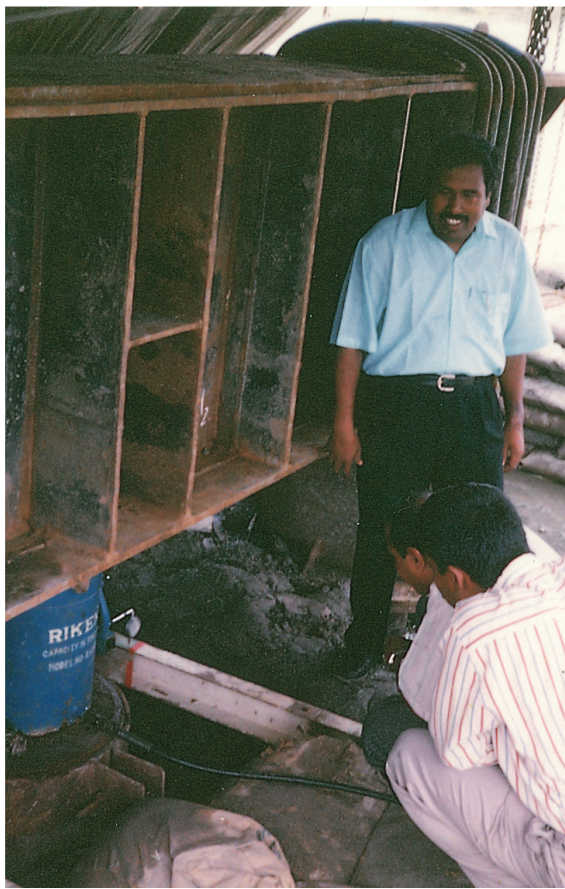
Static Load Test (220 ton) by applying anchor method.
