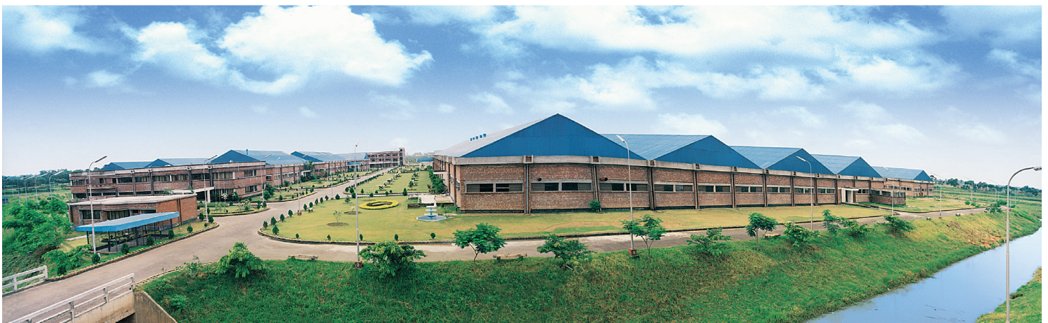
Shinepukur Ceramics Industrial Complex at Sarabo, Gazipur
