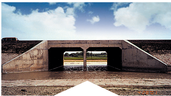
2 Vent Box-culvert in Jamuna Bridge Railway Link Project
