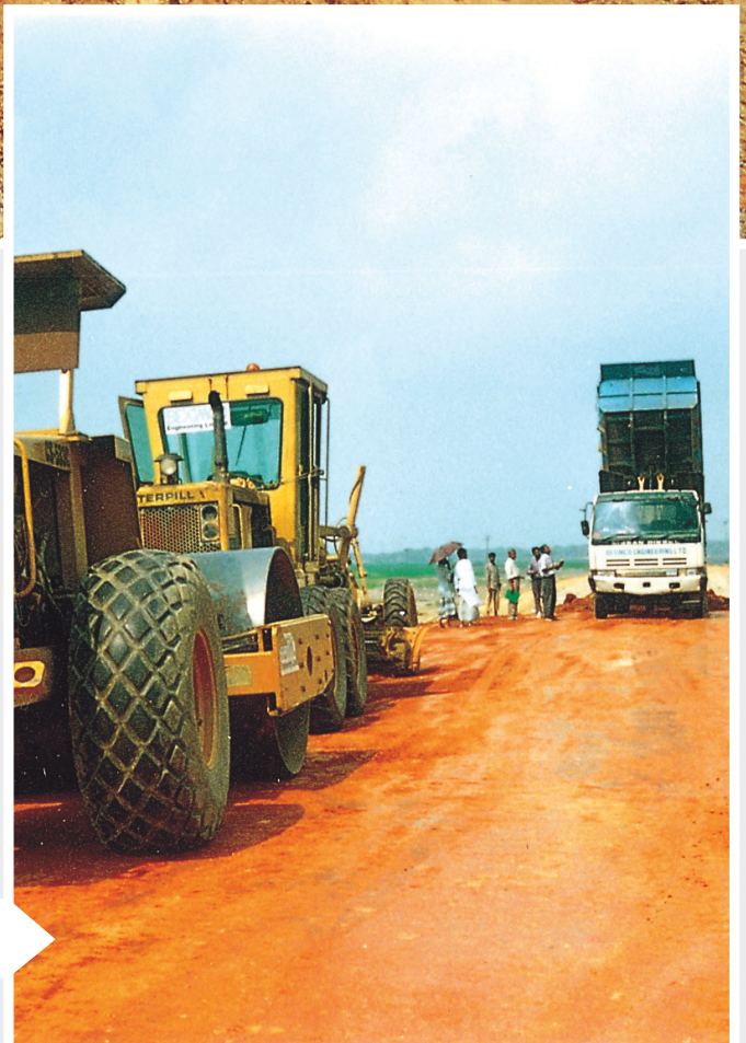
Construction of Railway Embankment, Jamuna Bridge Railway Link Project
