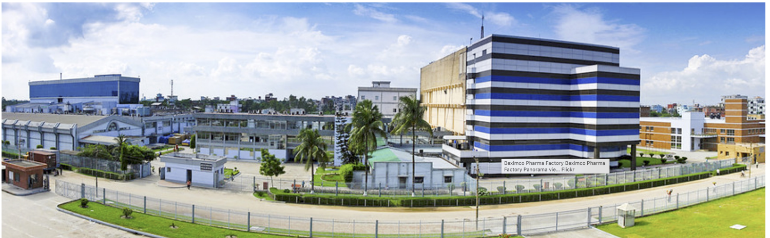
Production-Cum Office Building of Beximco Pharmaceuticals Ltd. at Tongi
