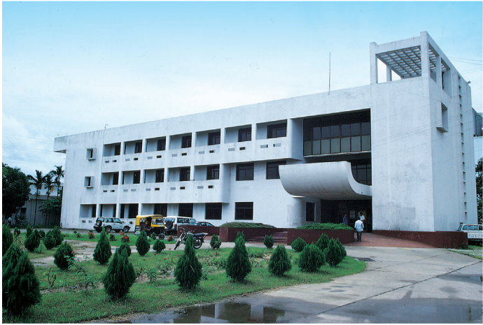
Administrative Building (3 storied of 2230 sqm. floor area) for 210 MW Chittagong Thermal Power Station at Raouzan, Chittagong
